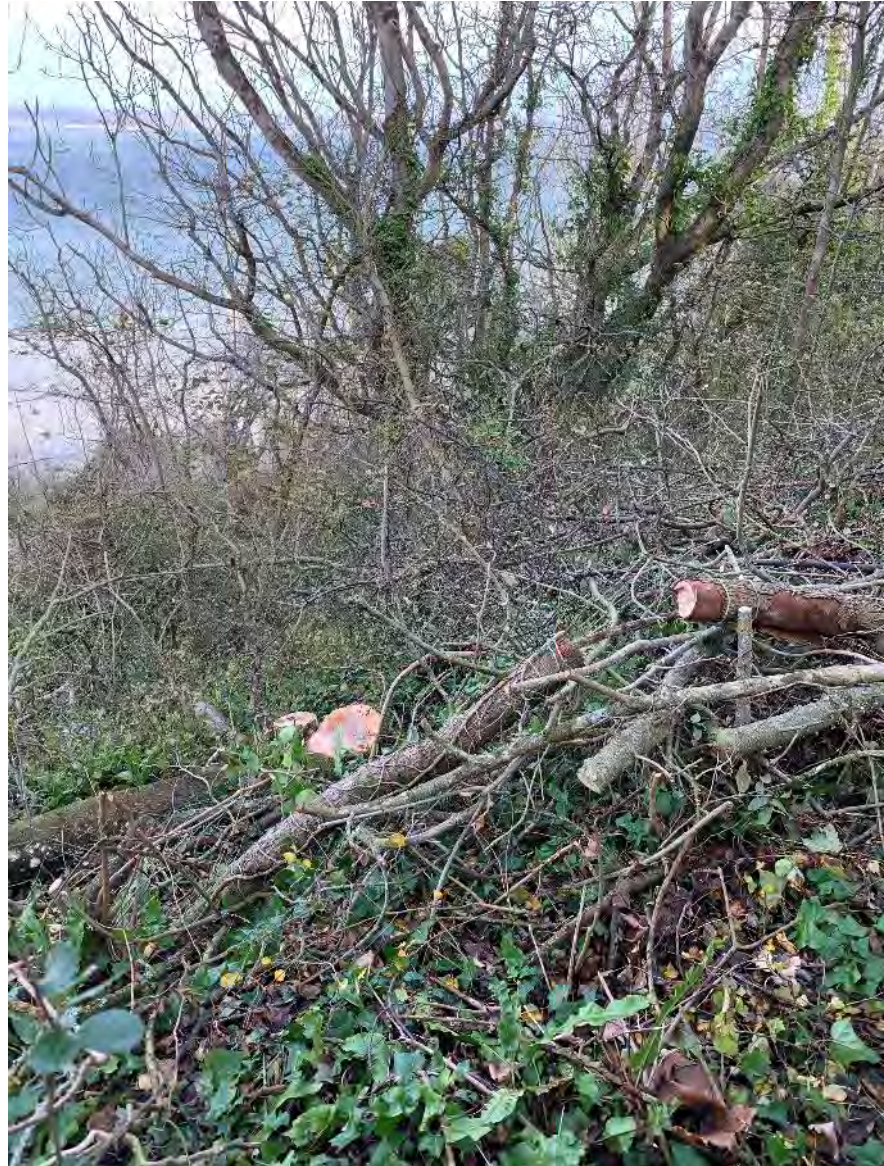
Line 65 IOW_5_S062 to 68/ Tree Works (1)
