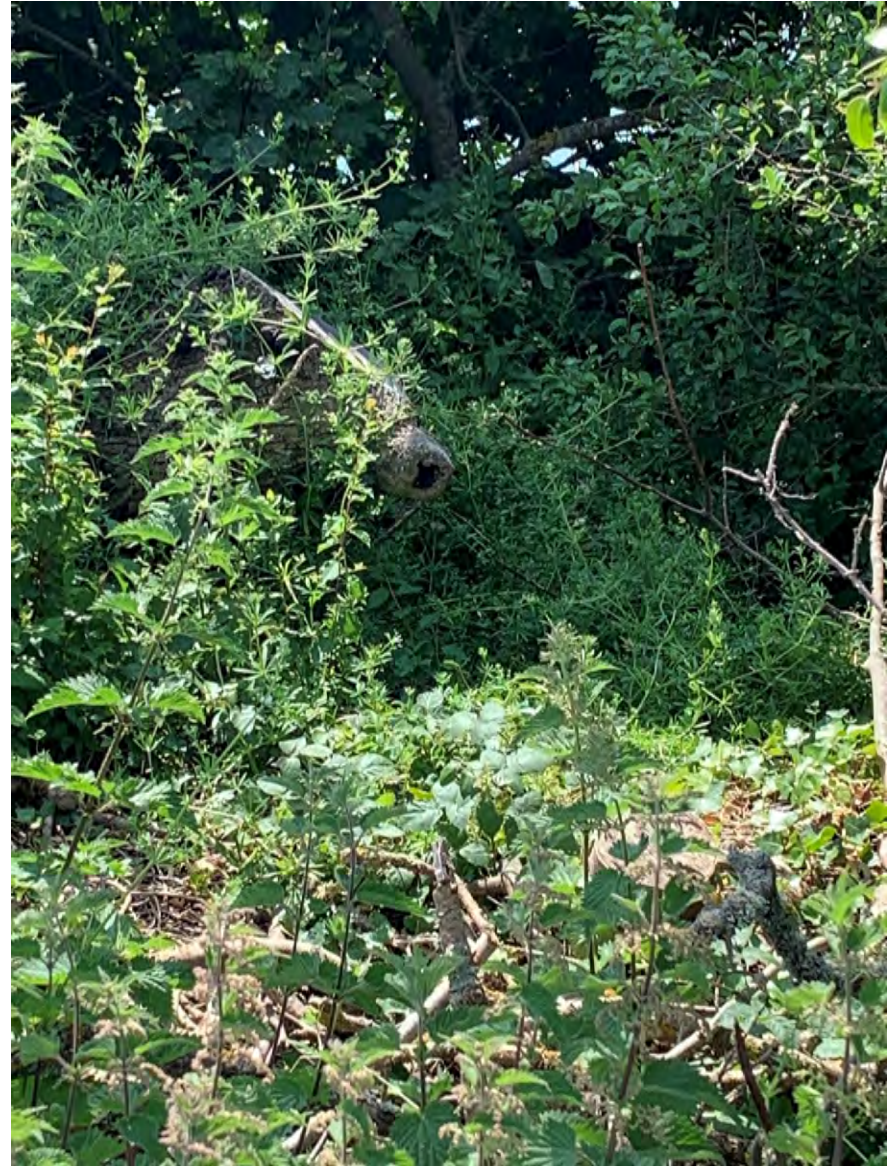
Line 51 IOW_4_S023 to S025/ Tree Works (1)
